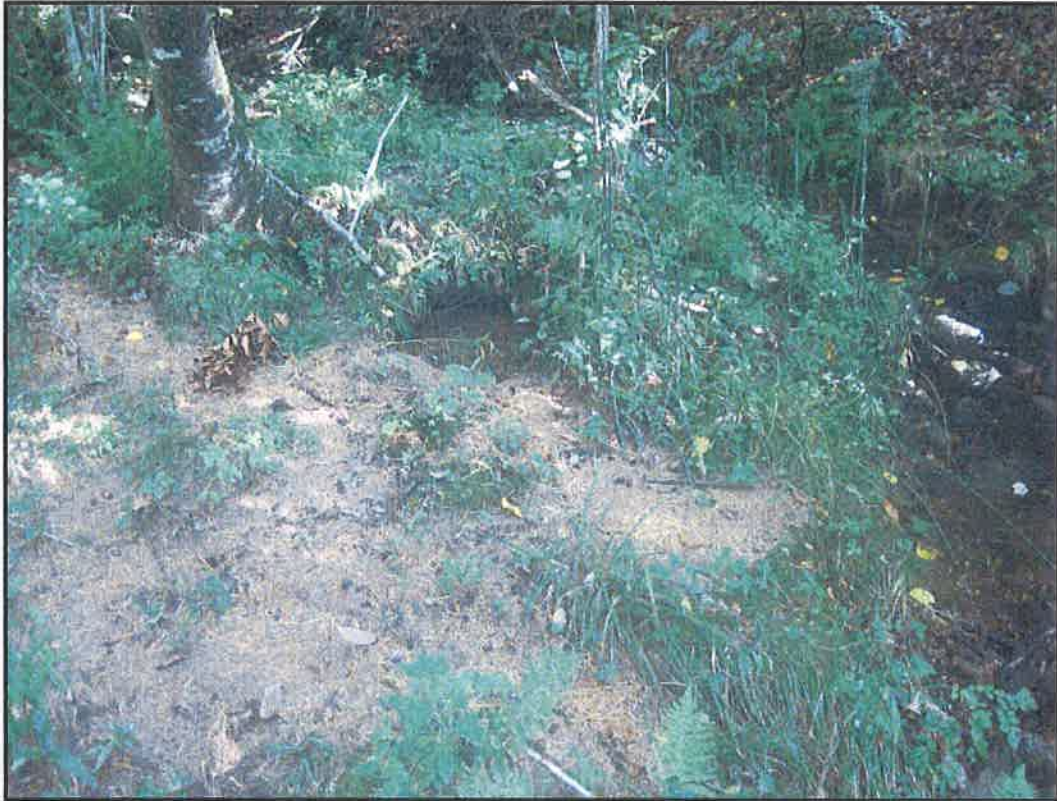
Sediment Area 4 at edge of stream: planted, seeded, and mulched, 9/22/14
