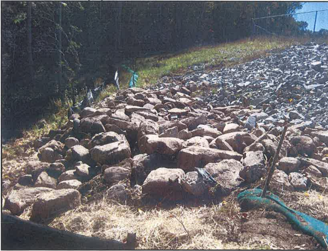
Reinforced splashpad above Sediment Area 5, 9/26/14
