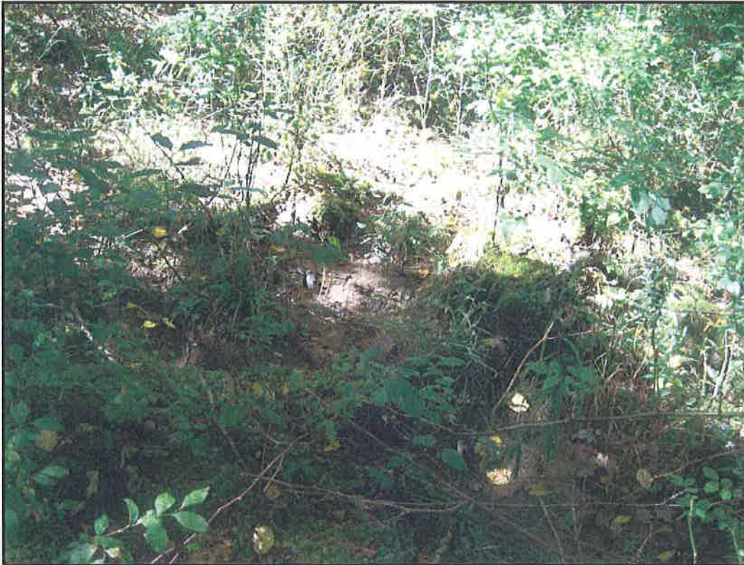
Sediment Area 2: well vegetated, seeded and mulched only, 9/26/14
