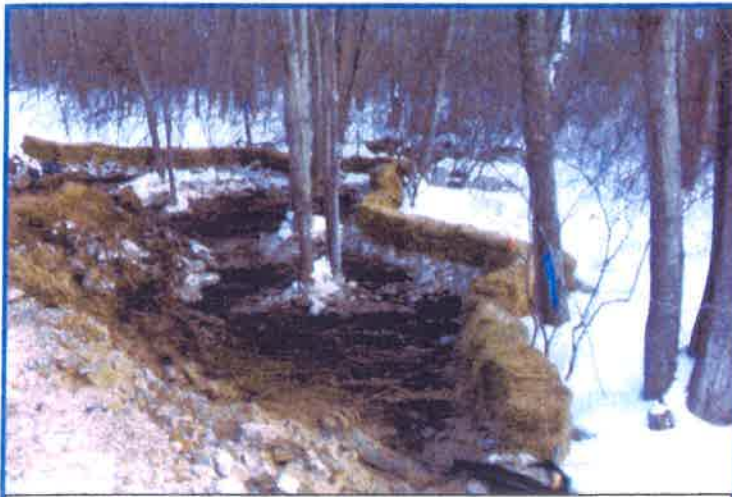
Final sediment removal condition in south side wetland
