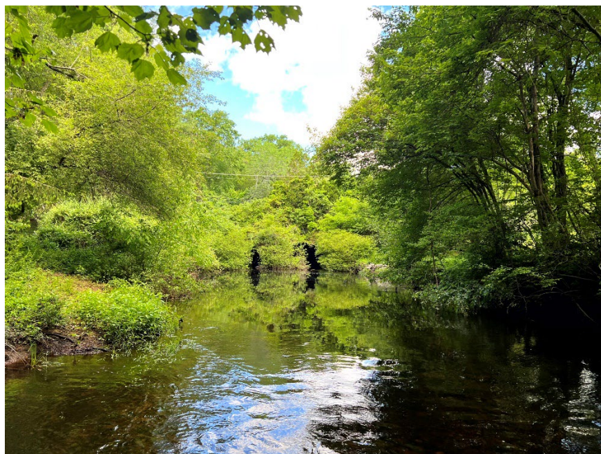
Looking north (upstream) at the bridge (May 2024)
