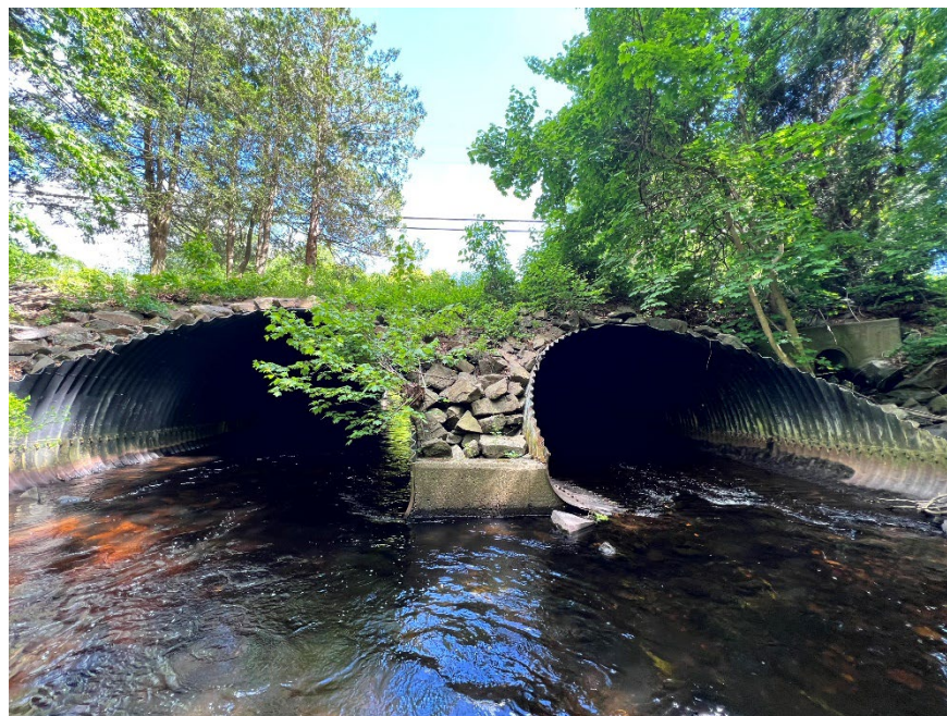
Looking south (downstream) at bridge (May 2024)
