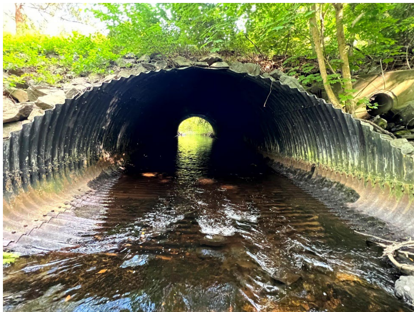
Looking south (downstream) at the bridge (May 2024)
