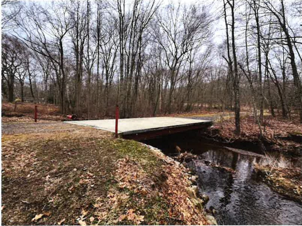
Photo 1: Site access bridge over Bride Brook
