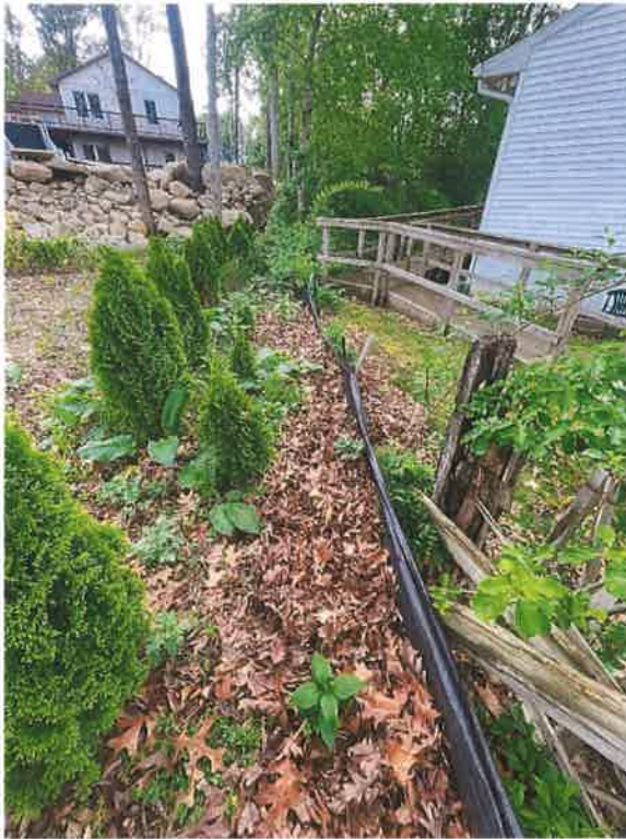
Figure 2: Eastern side of the fence failing due to sediment buildup.
