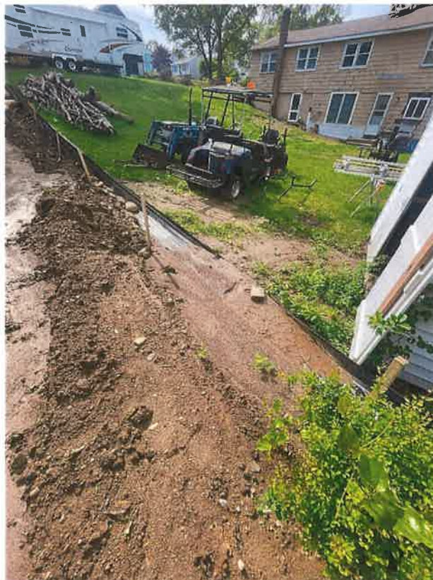
Figure 5: Silt visibly escaping through open northeast corner.
