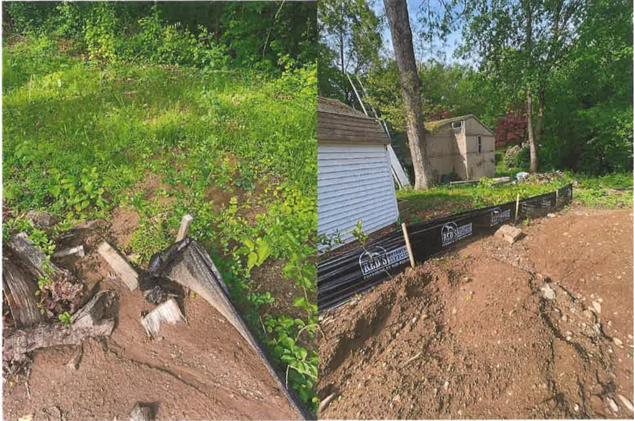
Figure 5: Silt visibly escaping through open northeast corner.
