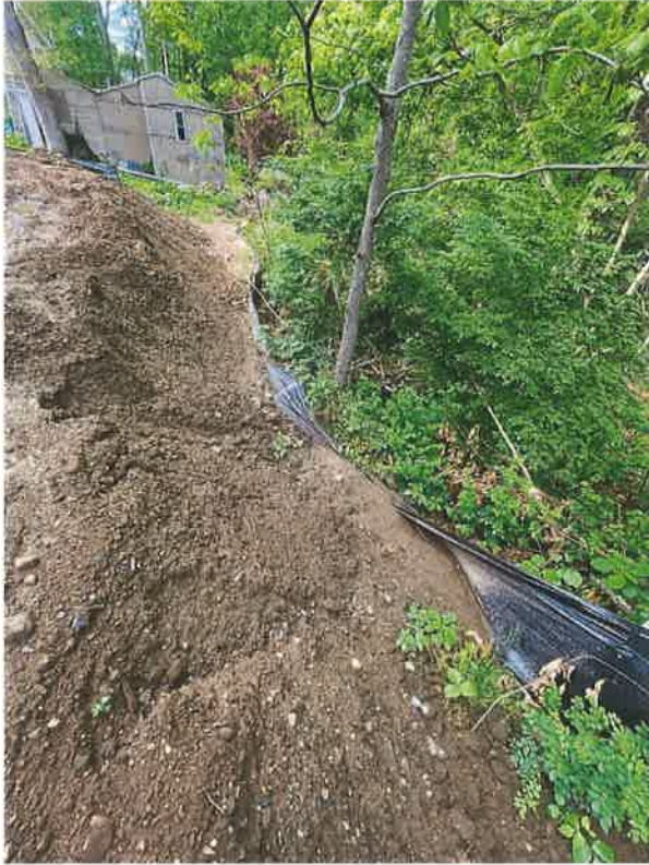
Figure 3: Second example Eastern fence section collapsing.
