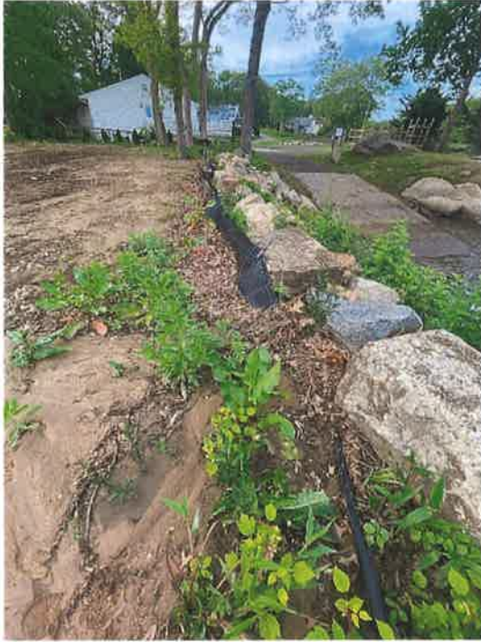
Figure 2: Eastern side of the fence failing due to sediment buildup.
