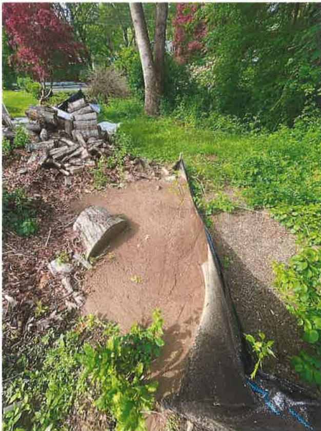
Figure 3: Second example Eastern fence section collapsing.
