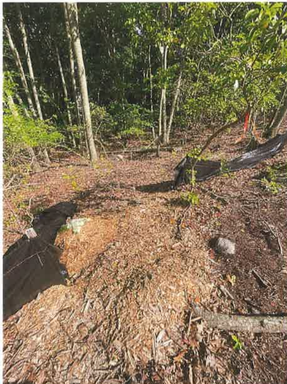
Figure 1: Failed Silt Fence.
