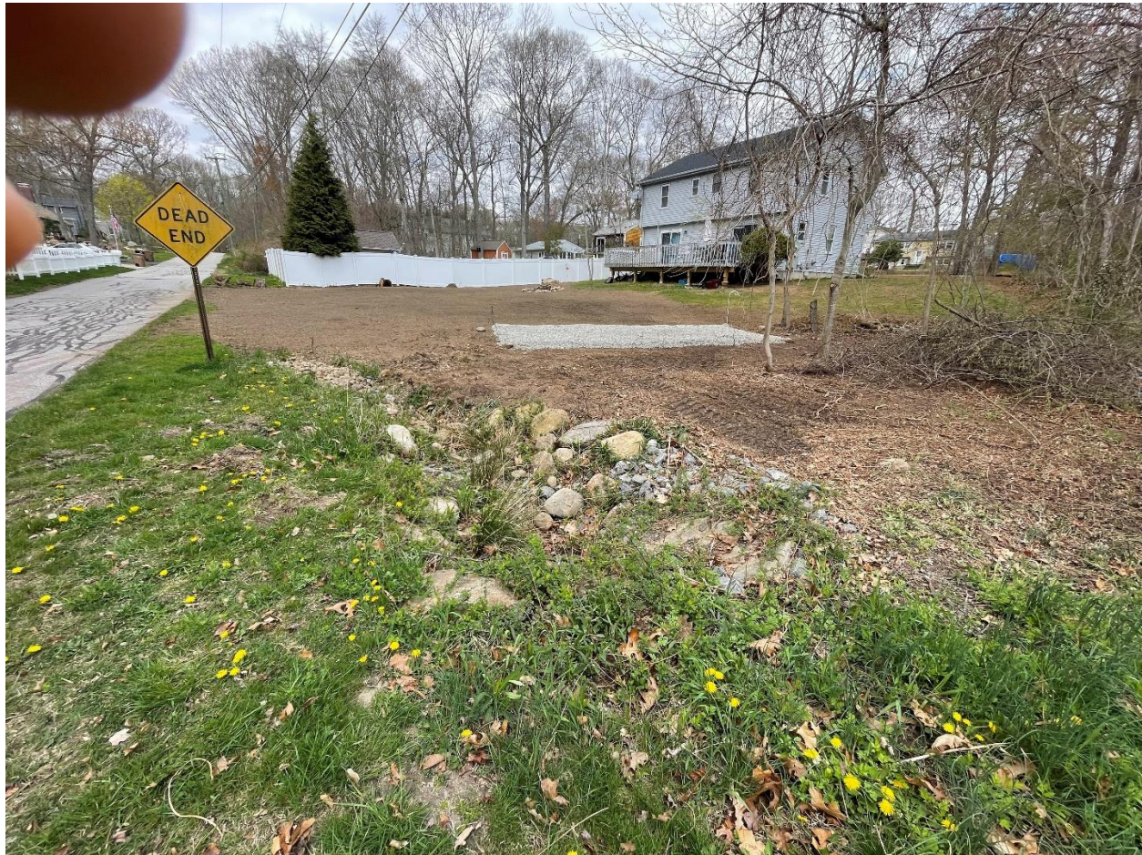
FIGURE 1 90-92 LAURELWOOD DRIVE - NOTICE OF VIOLATION
