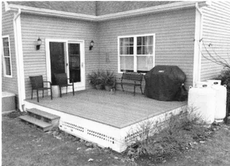
2 Knickerbocker Ln (Existing Deck)
