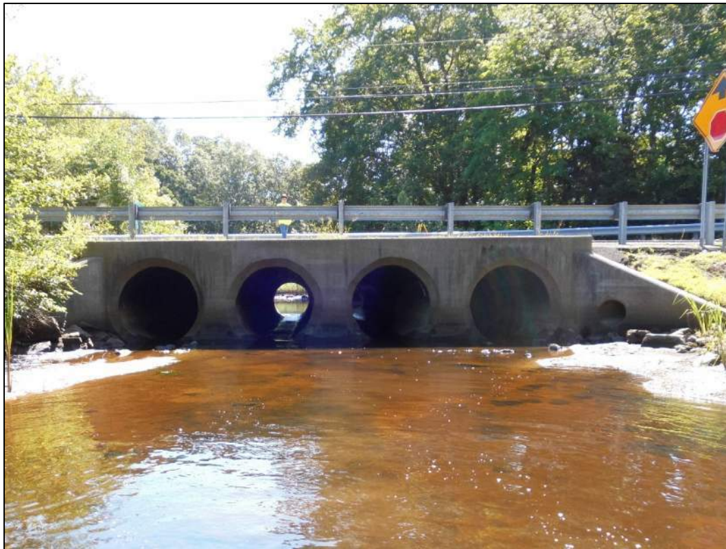
Photo No. 2 – West Elevation
