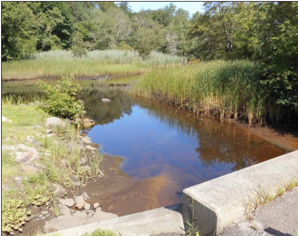
Photo No. 6 – Upstream from Bridge
