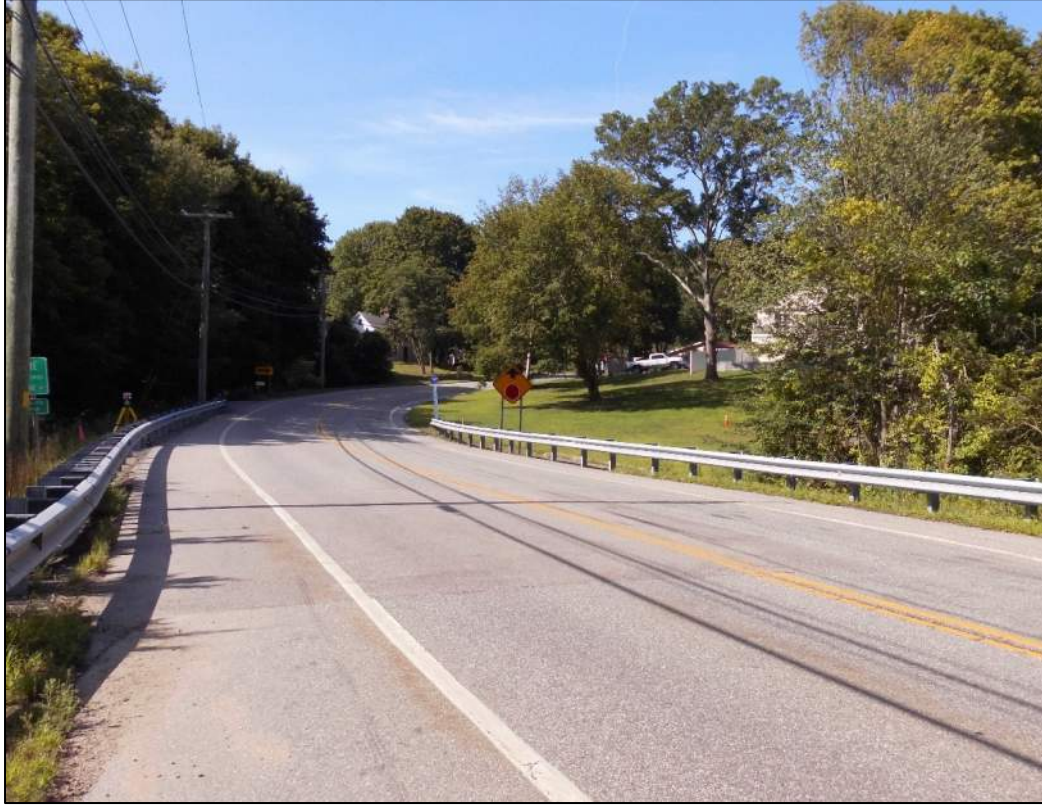
Photo No. 5 – Bridge from South Approach
