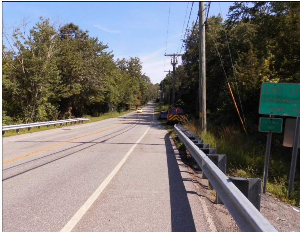
Photo No. 4 – Bridge from North Approach
