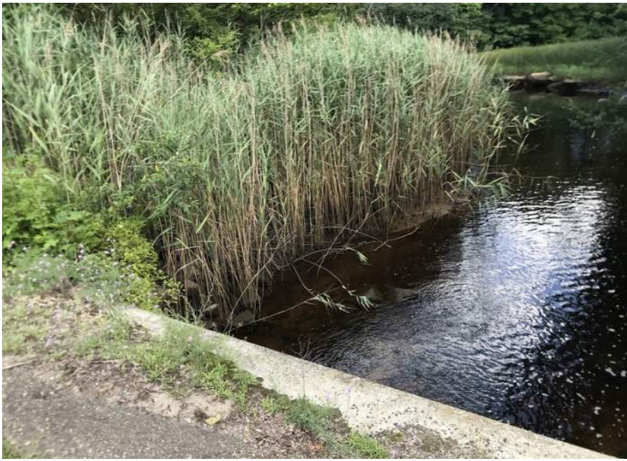
Looking southeast into tidal wetlands
