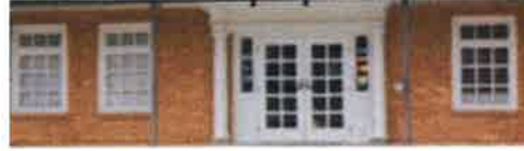
Greek revival entrance.
