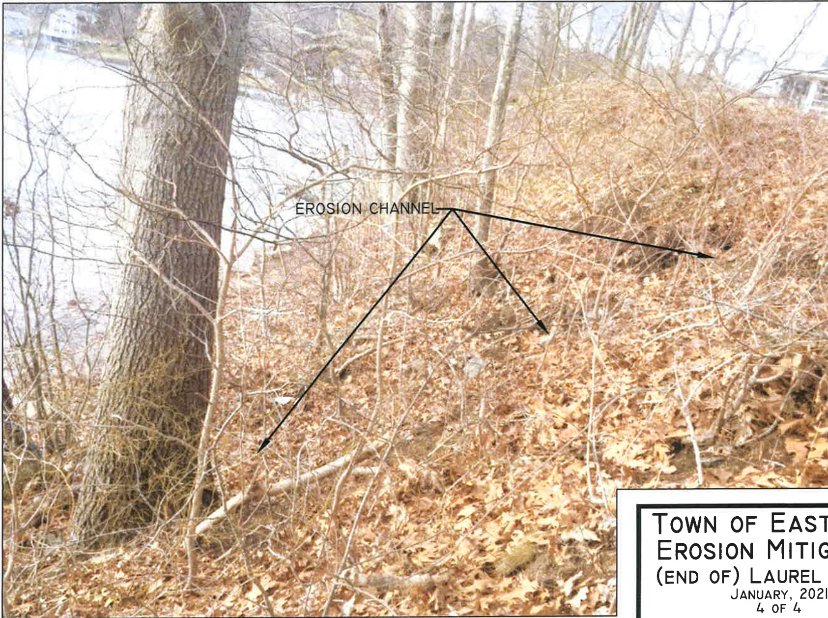
VIEW LOOKING NORTHWEST (PERPENDICULAR TO EROSION CHANNEL)
