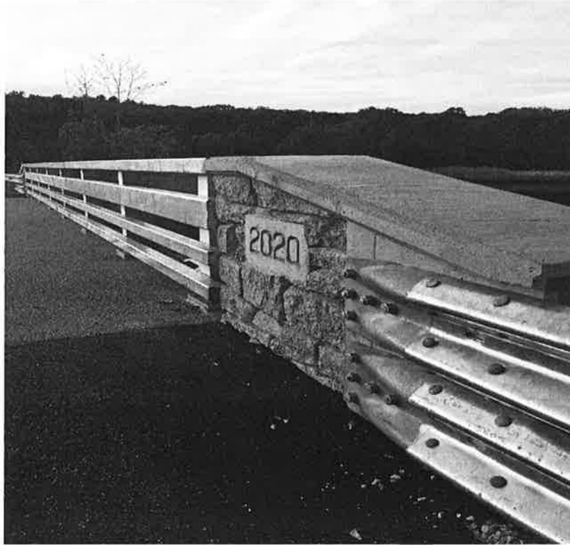
Photo by Tom Machnik - Mile Creek Bridge
