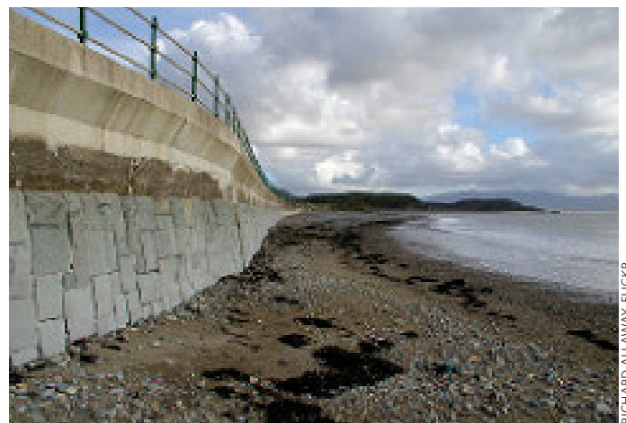
Erosion removes the natural protection provided by beach dunes and salt marshes and exposes hard structures to direct impacts and increased risk of structural failure.
