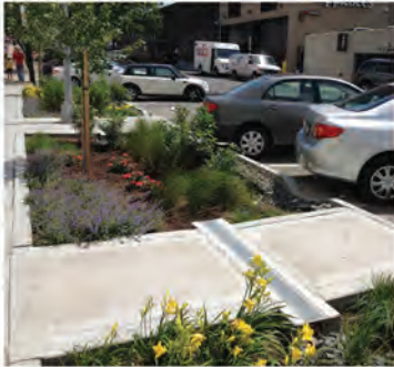
Curb-cuts funnel runoff to bioswales Photo credit: Chris Hamby
