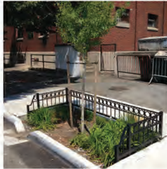
Curb-cuts direct runoff to street trees Photo credit: Chris Hamby
