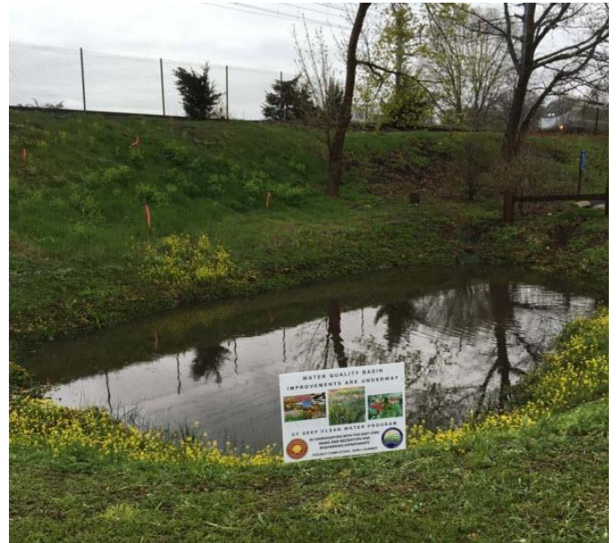
Detention Basin at Hole-In-The-Wall Outdoor Stormwater Classroom, Niantic. Source: Town of East Lyme.
