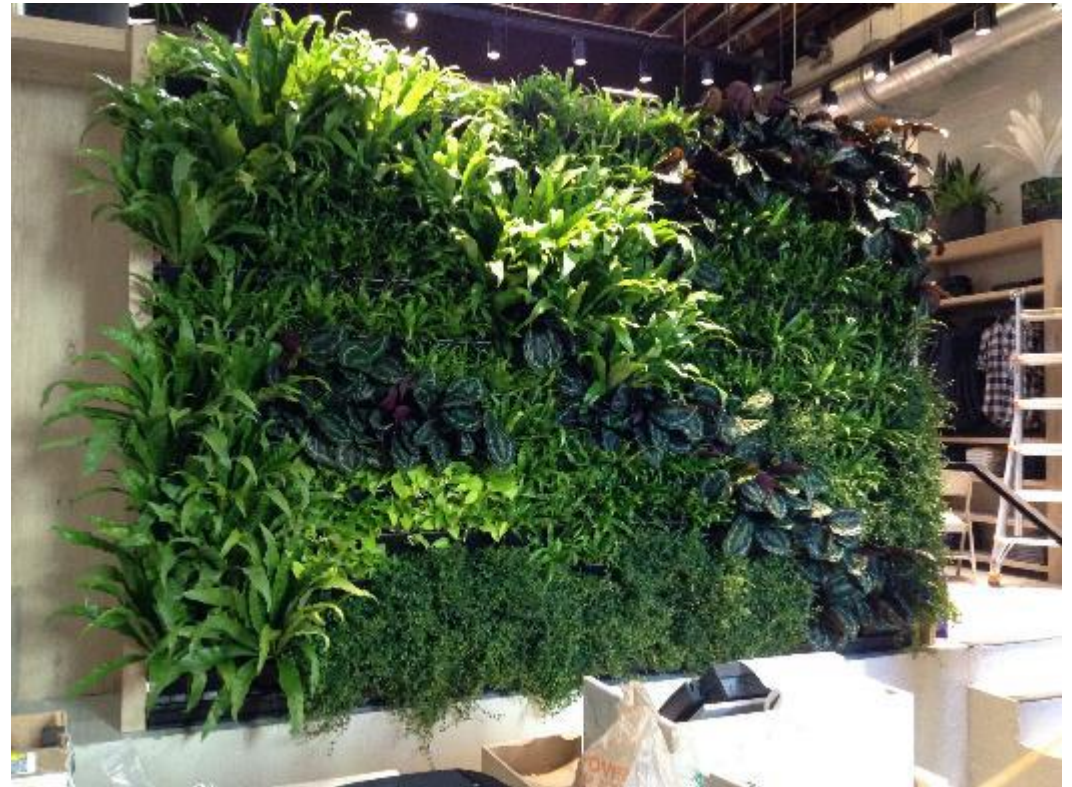
Green Wall installation at J Crew by seCTer client AgroSci of Colchester
