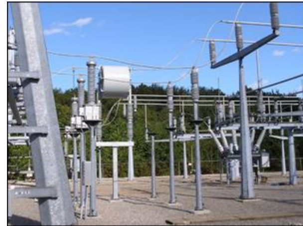
Groton Utilities, Buddington Rd. Sub-station
