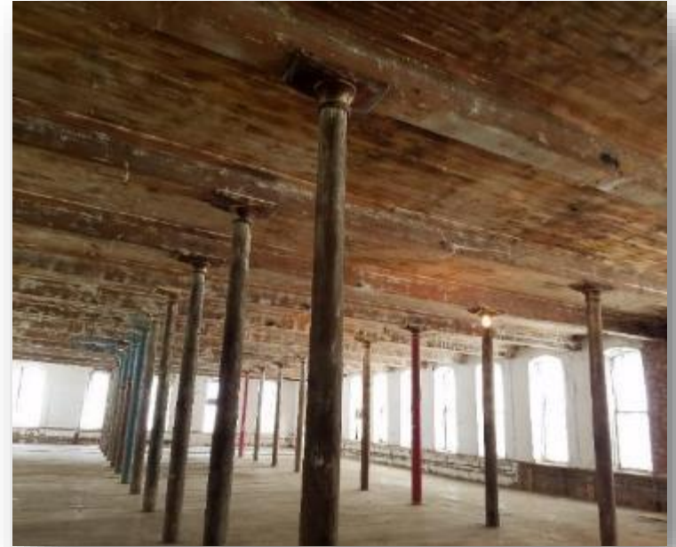
Early stages of renovation at Ponemah Mills, Taftville section of Norwich
