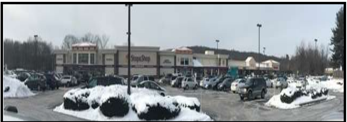
Figure 20: Stop and Shop
