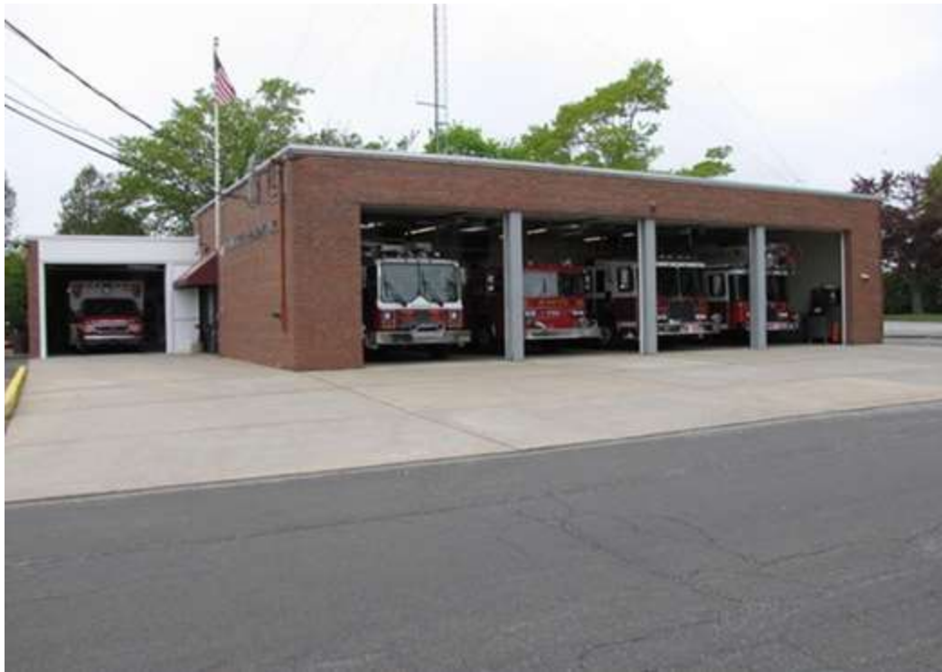
Figure 48: Niantic Station 1 Headquarters
