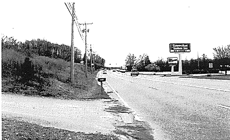
Existing view south on Route 161.
