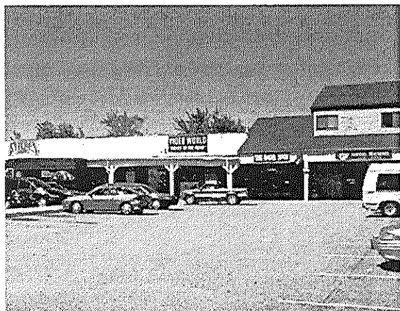
Existing condition at Midway Plaza on Route 161. Minor facade and sign improvements along with landscaping the parking lot would greatly improve the image of this stretch of the road.
