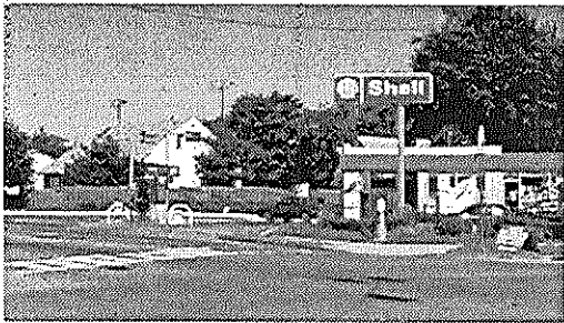
Existing condition of the Shell station at Flanders Four Corners.
