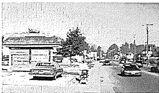
Existing condition along Pennsylvania avenue.
