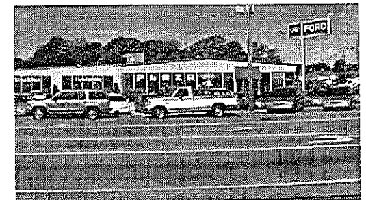
Existing conditions at the Ford Plaza. Trucks are parked out to the street edge on the green strip.
