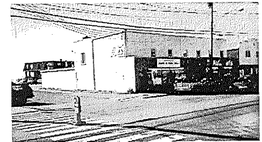
Existing conditions along Main Street.
