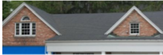
Visually interesting roof of a commercial building.
