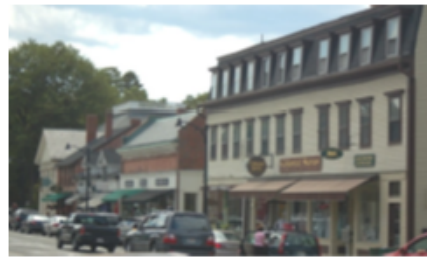
Vertically-aligned windows and entrances.
