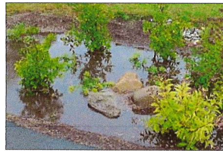
Rain gardens are built to hold water during rain events, however water should infiltrate the ground within 24 hours.
