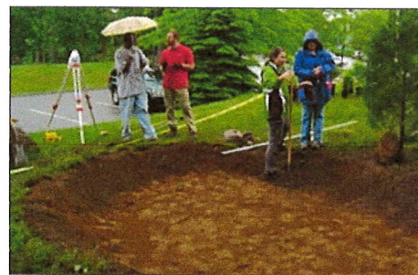
A berm can be created using soil excavated from the rain garden to accommodate for a sloping lawn.
