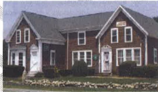
An example of a balanced and well-proportioned building.
