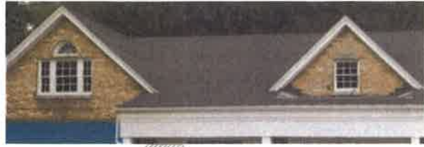
Visually interesting roof of a commercial building.
