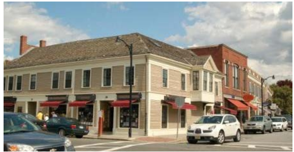
er building with attractive entrances and windows facing both major streets.
