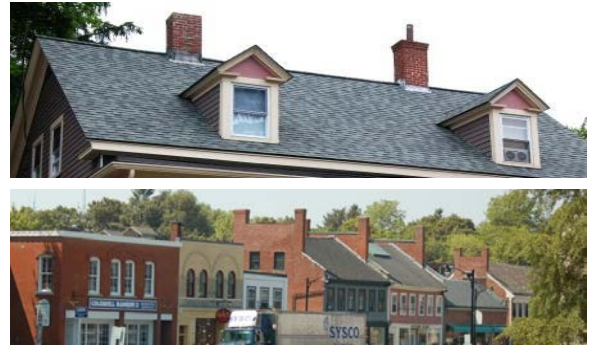
Vertically-aligned windows and entrances.
