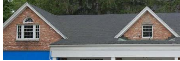
Visually interesting roof of a commercial building.
