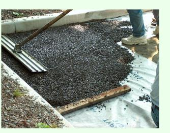
KBI FLEXI<sup>(R)</sup>—PAVE is a flexible, porous, weight bearing paving system alternative to traditional impervious asphalt pavement. This material is made from recycled tires and aggregate rock, bound together with moisture cure
