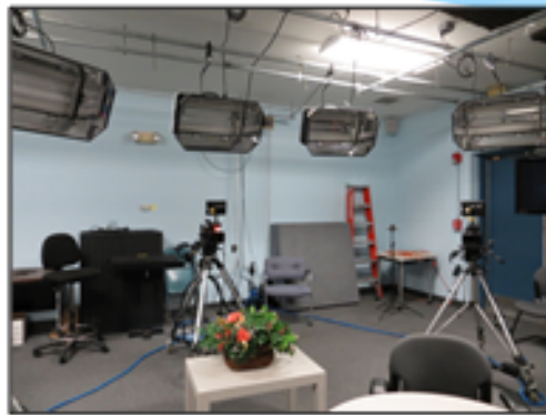
LED lighting grid in-studio COMPLETED
