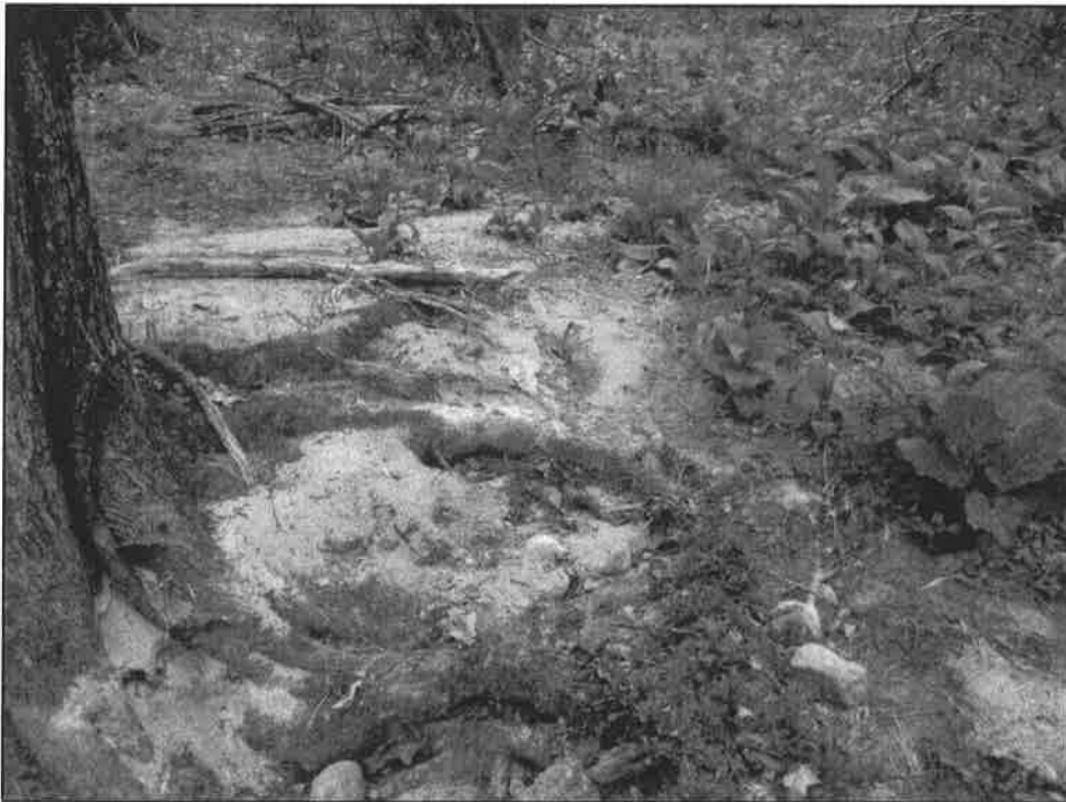
West sediment deposit at mouth of the tributary, 5/13/14
